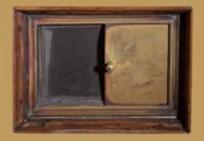
The heating of the castle was provided not only by fireplaces and tiled stoves, but also by several boilers located in the basement. The rooms on the ground floor and the first floor were heated in this modern way. The heating was based on the principle of heating the air, which was distributed through shafts in the walls of the castle. On the sides of the fireplace are brass doors through which warm air flowed into the room.
